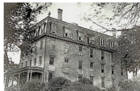
AS PRESIDENT OF VILLANOVA COLLEGE (1878-1880), FR. FEDIGAN ADDED A FOURTH FLOOR AND ENLARGED THE OLD BELLE-AIR MANSION. PICTURES ABOVE SHOW BEFORE AND AFTER RENOVATIONS.
