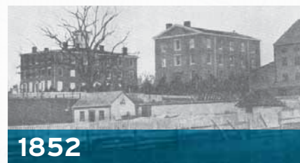
1852 RENOVATIONS OF THE BELLE-AIR MANSION AND THE FIRST WING OF THE COLLEGE (NOW THE EAST WING OF ALUMNI HALL) ARE COMPLETED. THE MANSION WAS DESTROYED BY FIRE JANUARY 10, 1912.
